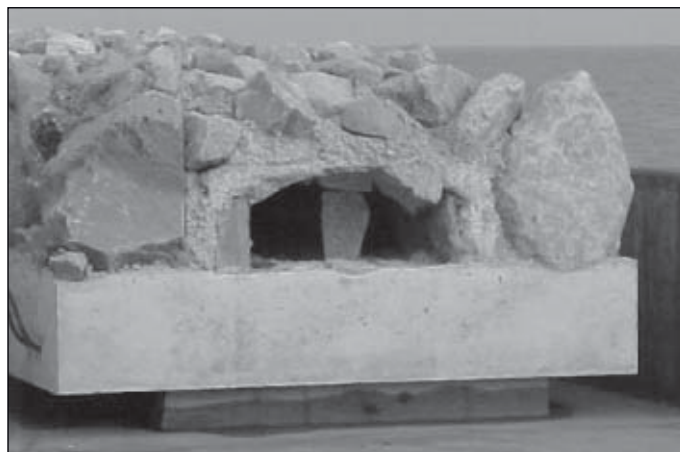
Gulfstream used prefabricated reefs such as this (left) to provide seafloor replacement environments (right) for epiflora, epifauna, and fish disturbed by its pipeline construction (Fig. 1).
